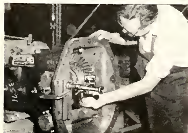
Precision dial indicator registers backlash in transmission and differential gears. This operation is quality controlled to a thousandth part of an inch.
