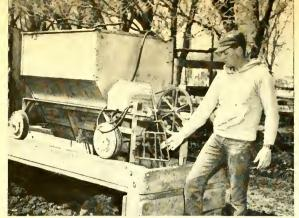
This rod in Otto Geiger's right hand reverses the automatic feed wagon to return it as soon as it reaches the end of the feed bunk.
