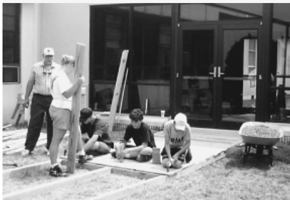
One of the surfaces students constructed within the hospital courtyard included wooden decking.
