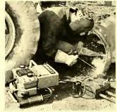
L. New low-cost portable air-cooled gasoline-engine-driven welder can be carried anywhere for construction and maintenance welding. Weighs 55 pounds. (Hobart Bros.)
