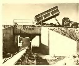
Salt is removed from "garden ponds" and trucked to these hoppers where the big conveyer belts move it to storage.
