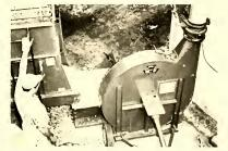
T. A crop blower designed for "drive-by" filling of the tallest silos. Operator can unload fast, pull straight ahead, and then get back to the field. (Massey-Ferguson)
