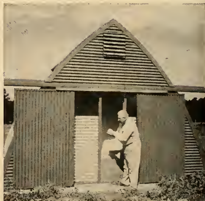
This Quonset 16, equipped with a drying fan and tunnel, lets Fisher store and dry his soybeans, wheat, oats or corn without worrying about loss of any of the grain from moisture. He's looking at some of the 1,500 bushels of wheat harvested this year, now under seal at support price. He parks tractors in the building when it's empty.
