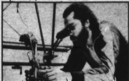
Geography major Semeret-AB-Chernet operates the department's new stereoplotter, which projects a three-dimensional image from aerial photographs into the viewer.
