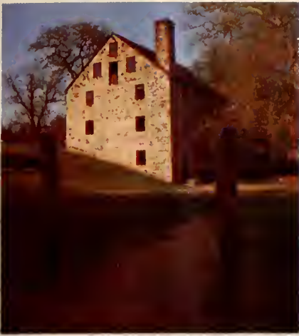
Washington's restored grist mill.
