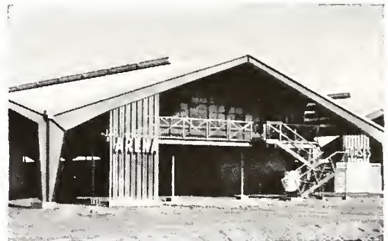
The mezzanine dormitory for exhibitors is neatly tucked under the weathersealed Butler metal roof — creates a modern, functional appearance that is strikingly distinctive.
