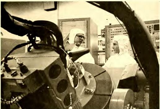
Making the inertial guidance systems for the Apollo mission is a big responsibility. More than two hundred tests are performed on every system before it goes into an Apollo vehicle. Some of these tests go the full distance. All 600,000 miles. These flight simulations include the initial shock of launch, directional changes, temperature extremes, space radiation effects, vibration produced by aerodynamics and the rocket's engines, even the shock of landing.
