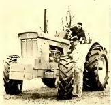
D. Up to 30 percent of the tractor's drawbar horsepower is available through this hydrostatically-driven front wheel D21-11 four-wheel-drive tractor. (Allis-Chalmers)
