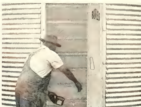
Easy sampling, bagging. Mr. Miller takes a wheat sample through convenient Butler bagging and sampling port. Die formed door boards are grain-tight.
