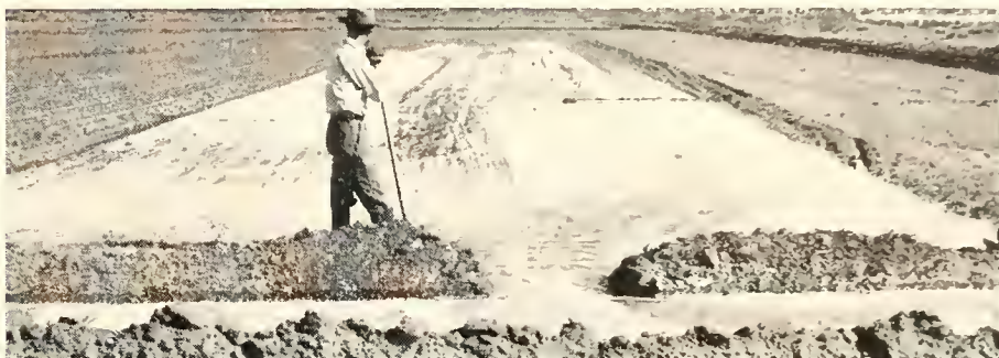
The even spread of water on this field proves that a good job of leveling had been done. Oats were planted before the water was allowed to enter the field.
