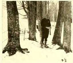
Andy carefully installs plastic pipeline to sugar maples. Sap flows gravity through tap and pipeline to storage tank.
